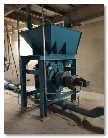
Figure 4: The new Kreisel rotary valve
