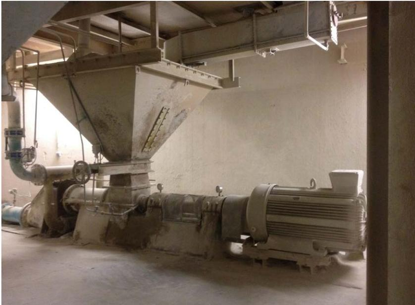
Figure 3: The old screw pump
